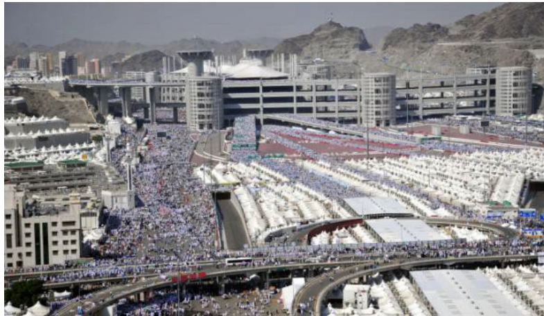
Figure 2-2: Aljamarat Bridge. Source: Edrees (2016).
